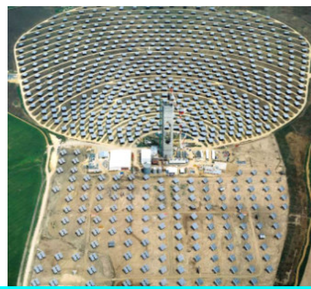
11 MW Solar Power Tower, Spain
