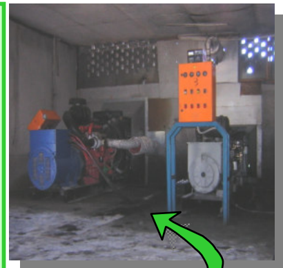
A 150 and 350 kW diesel generator at Tsumkwe
