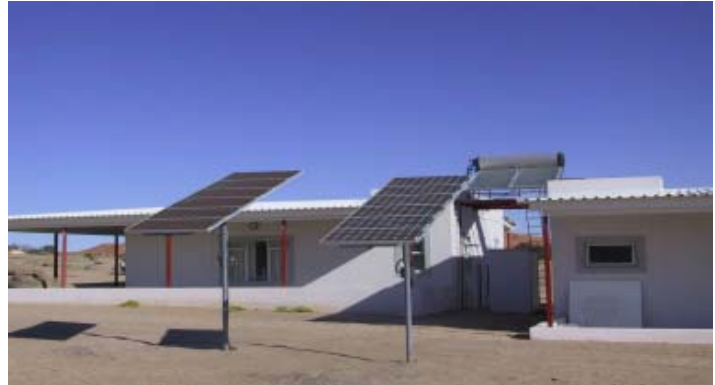
Newly erected buildings at the Gobabeb Centre were designed to make optimum use of renewable energy, as these solar panels demonstrate.
