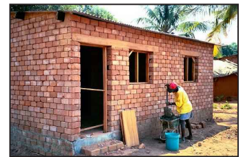
Fired clay brick (an energy intensive resource) building under construction
