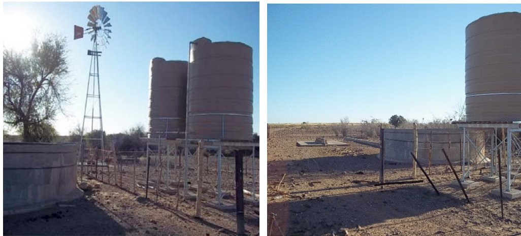
Figure 2 The layout of the infrastructure around the water point: a non functional windmill, water tanks, a farm dam and a livestock watering trough in the background (second picture). The fence around the water point has collapsed and is not maintained.
