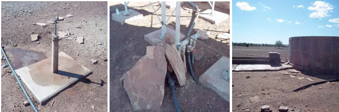
Figure 1. The water infrastructure at Khaitsub farm. The middle picture shows some of the measures taken by the community members to protect the infrastructure. In all the pictures it clearly shows the extent of exposed water pipes.
